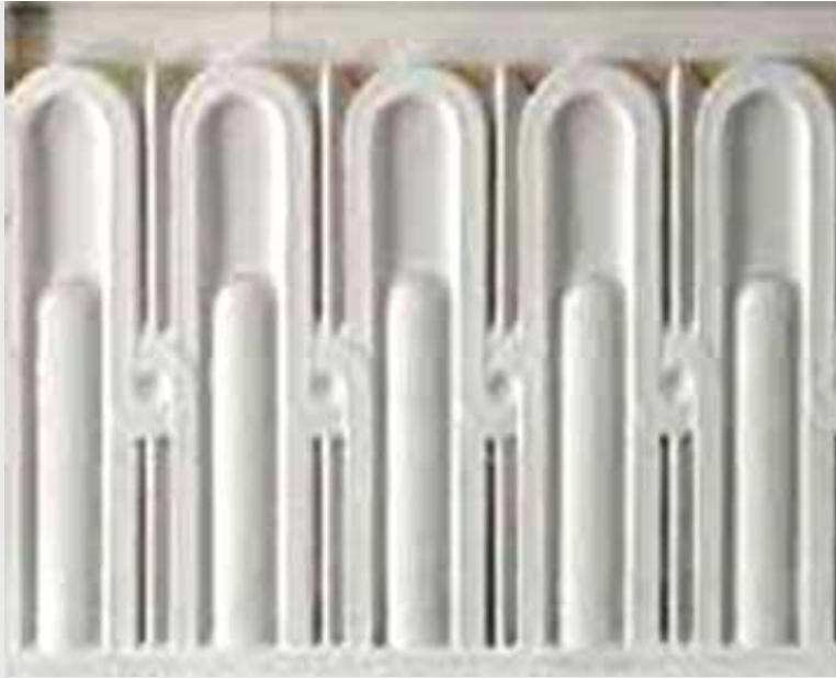
Example, fireplace frieze: Risman House
