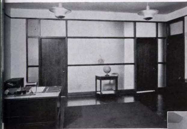
ABOVE: A bright, attractive office is screened from the reception room in the offices of the E. J. Hunt Company, Detroit. The glass is double-glazed Louvrex with Satinol finish on the outside to absorb reflection.
