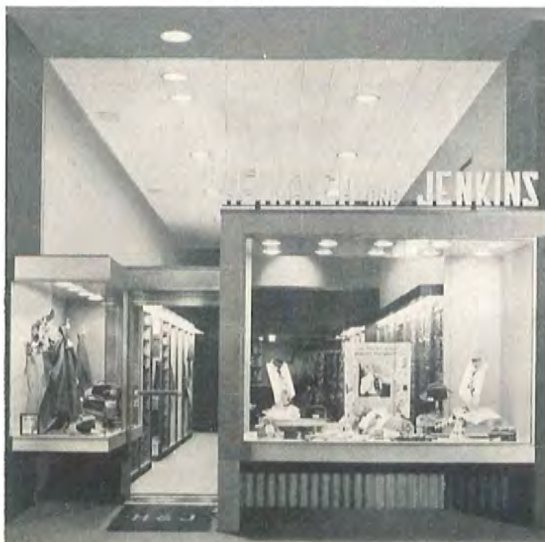
Location: Cumberland, Md. Architect: S. Russ Minter, Cumberland. Products Used: Carrara Structural Glass; Pittsburgh Polished Plate Glass; Herculite Tempered Plate Glass Door; Herculite Door Frame Assembly; Pittco De Luxe Store Front Metal.
