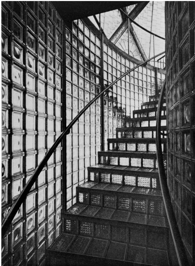
Figure 9 - Interior staircase of the Glass Pavilion, 1914 (photo from Wikimedia Commons)
